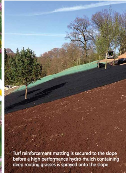
Turf reinforcement matting is secured to the slope before a high performance hydro-mulch containing deep rooting grasses is sprayed onto the slope
